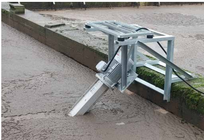
TurboStar® mixer on standard mounting bracket
