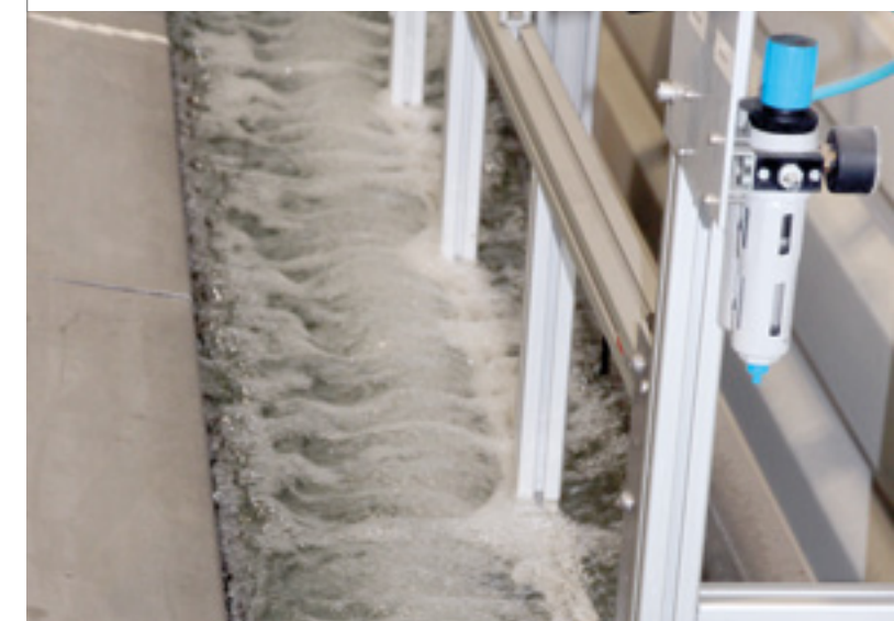
Quality inspection of an INVENT aeration system
