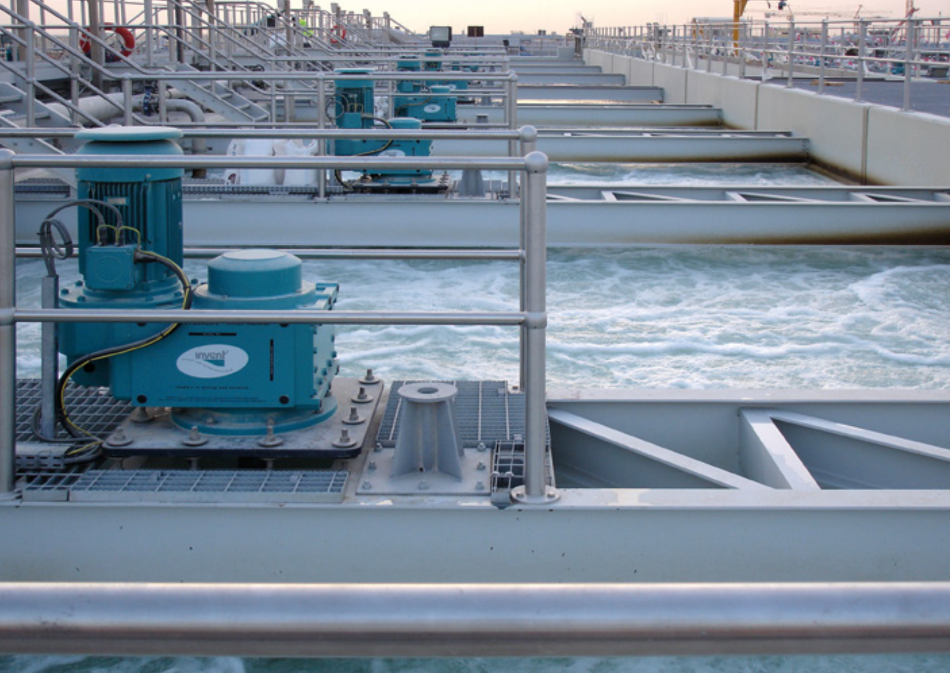
HYPERCLASSIC® -Mixing and Aeration System in a municipal wastewater treatment plant
