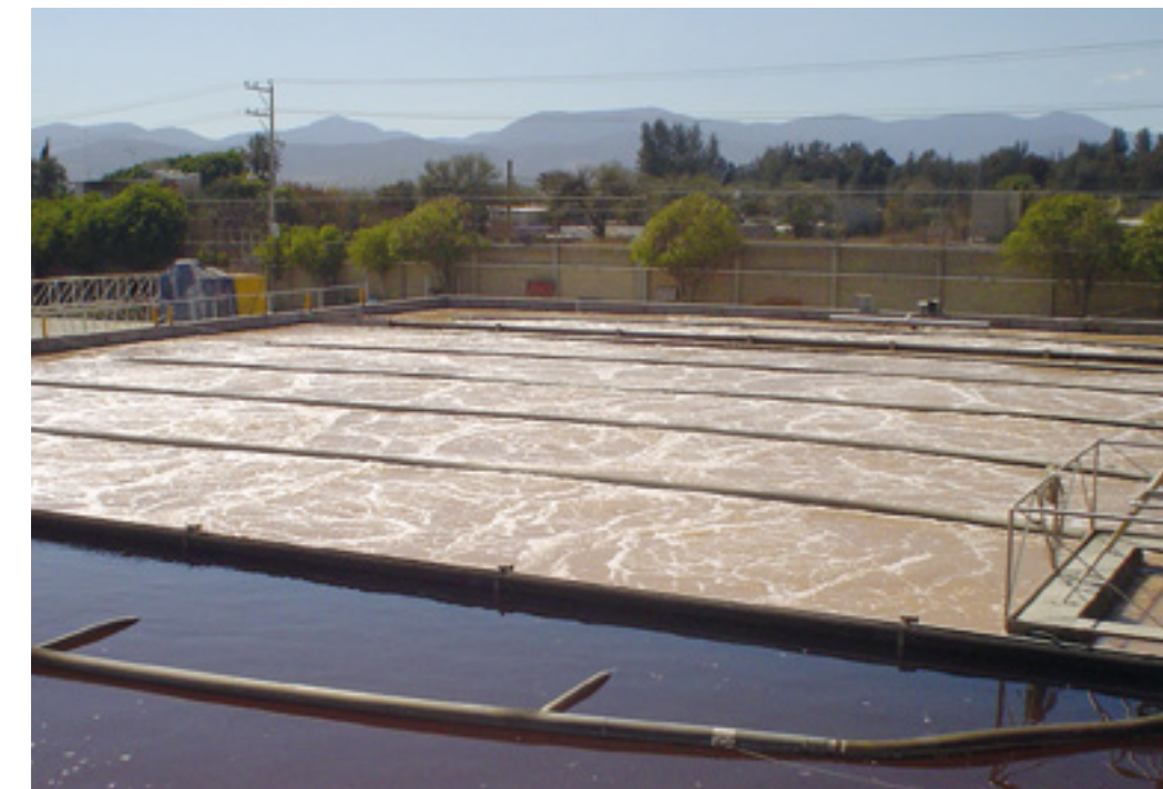
E-FLEX®-FLOAT Aeration System in operation in an activation basin
