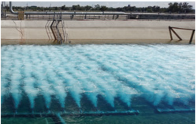
WWTP Westdale, WA, Australia
