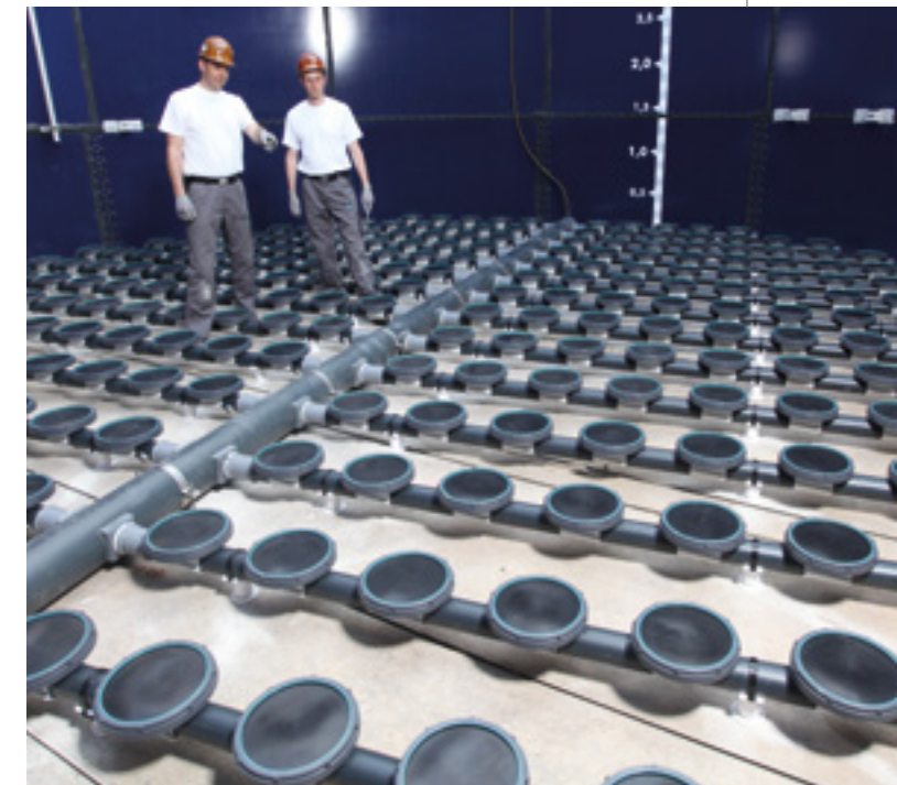
Installation of the iDISC® Membrane Aeration System
