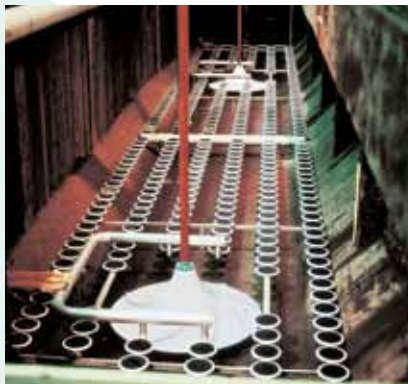
2 out of 48 HYPERCLASSIC® -Mixers in a wntp in Stockholm, Sweden
