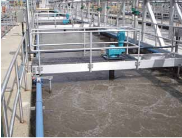
3 out of 90 HYPERCLASSIC® -Mixers in the wntp Bowery Bay, New York, USA
