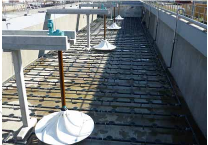
4 INVENT HYPERCLASSIC® -Mixers combined with iDISC® Membrane Aeration System
