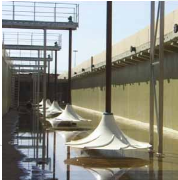
6 out of 120 HYPERCLASSIC® -Mixers in a wtp in Berlin, Germany
