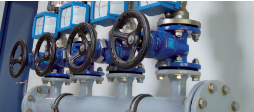
Drinking water treatment plant Luisenthal, Germany 35 VAG BETA® 200 Gate Valves
