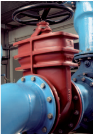
Schwetzingen Waterworks, Germany 10 VAG BETA® 200 Gate Valves
