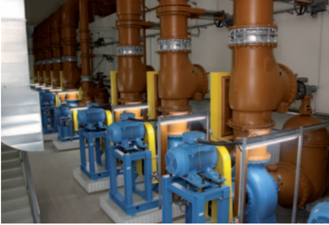
Cologne combined pumping station Rodenkirchen, Germany 6 VAG KOS Gate Valves
